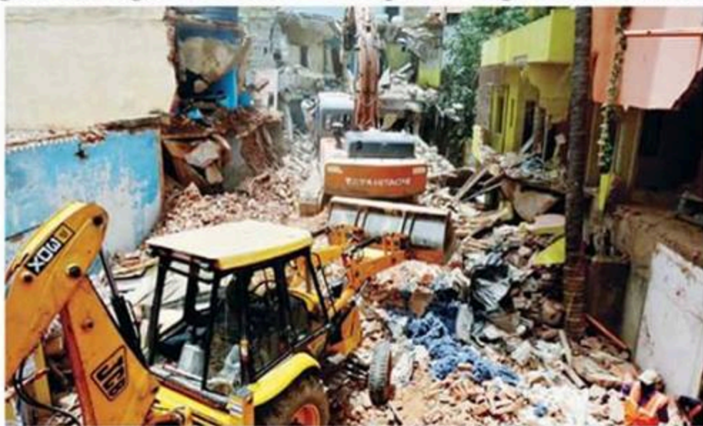
BBMP's recent demolition drive in Dodda Bommasandra
